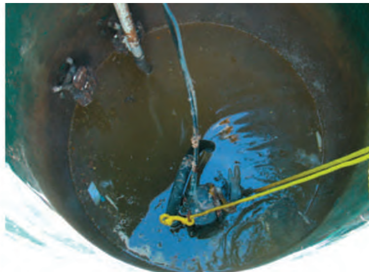
Top view showing Upgrade retrofit.
